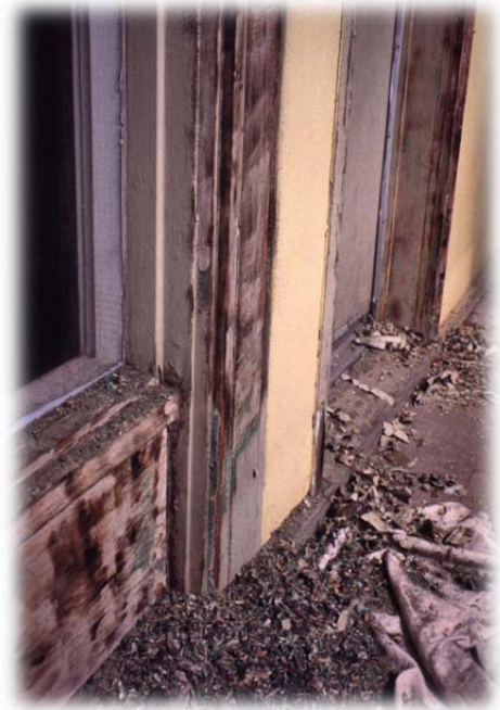
Image: This photograph reveals lead paint scrapings on a floor. Source: CDC/ Aaron L. Sussell
